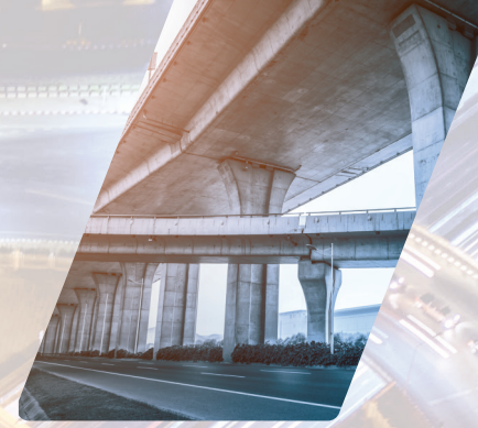
Culverts and Bridges construction
