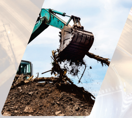
Earthworks (excavation, filling, leveling, etc.).
