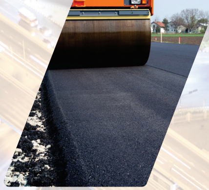
Paving and asphalt works.
