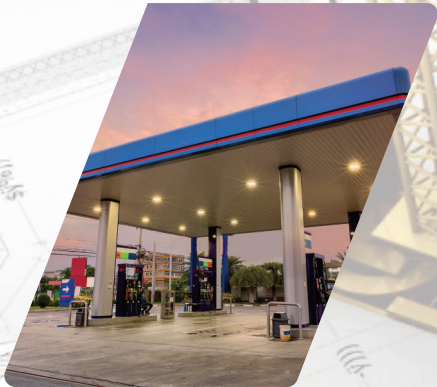
Fuel station development.
